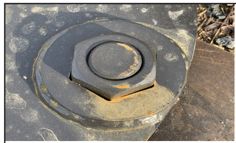
Figure 4.7b Bolt Thru Nut
